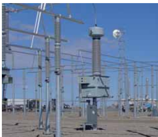
4. 245 kV Inductive voltage transformer. Coyote Switch (USA).
